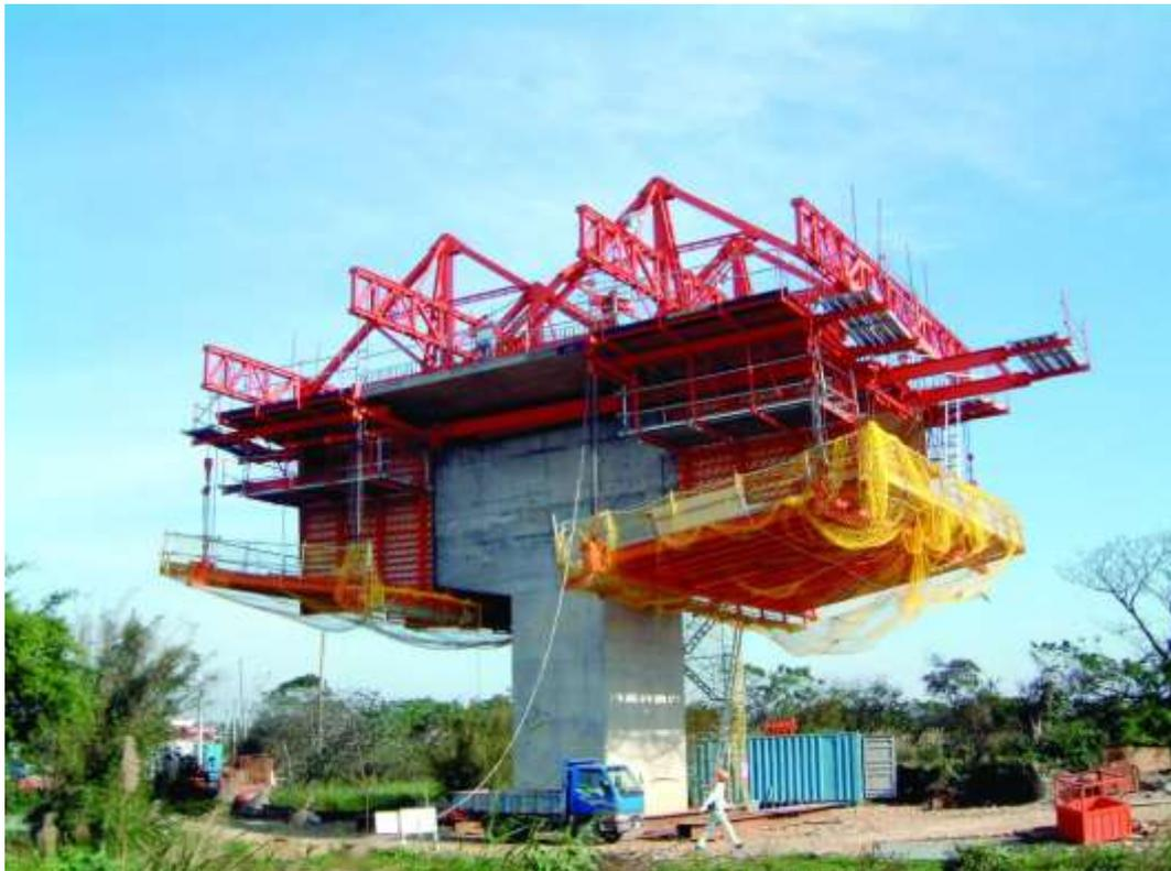
Stability of the end cantilever is maintained by using temporary pier supports as the end span is begun. On the western side the end span will tie into a pier (Pier F), as shown above in **Figures 2.7** and **2.8**. On the eastern side the end span will tie into the retained embankment with culvert openings as shown below in **Figures 2.11** and **2.12**.
